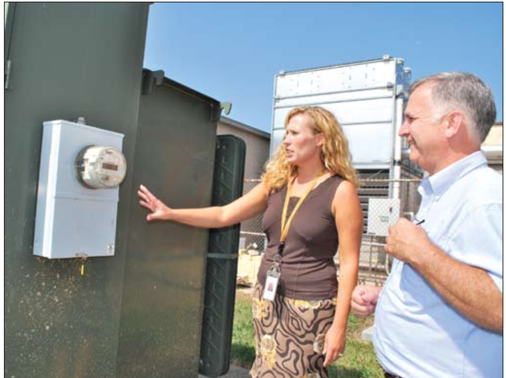
Jon Nipple, energy manager with the School Energy Managers Project, and Molly McComas, the point person for the project in Williamstown Independent Schools, check a main meter on the district's campus. Changing the type of rate on that meter will save the district $30,000 per year.
